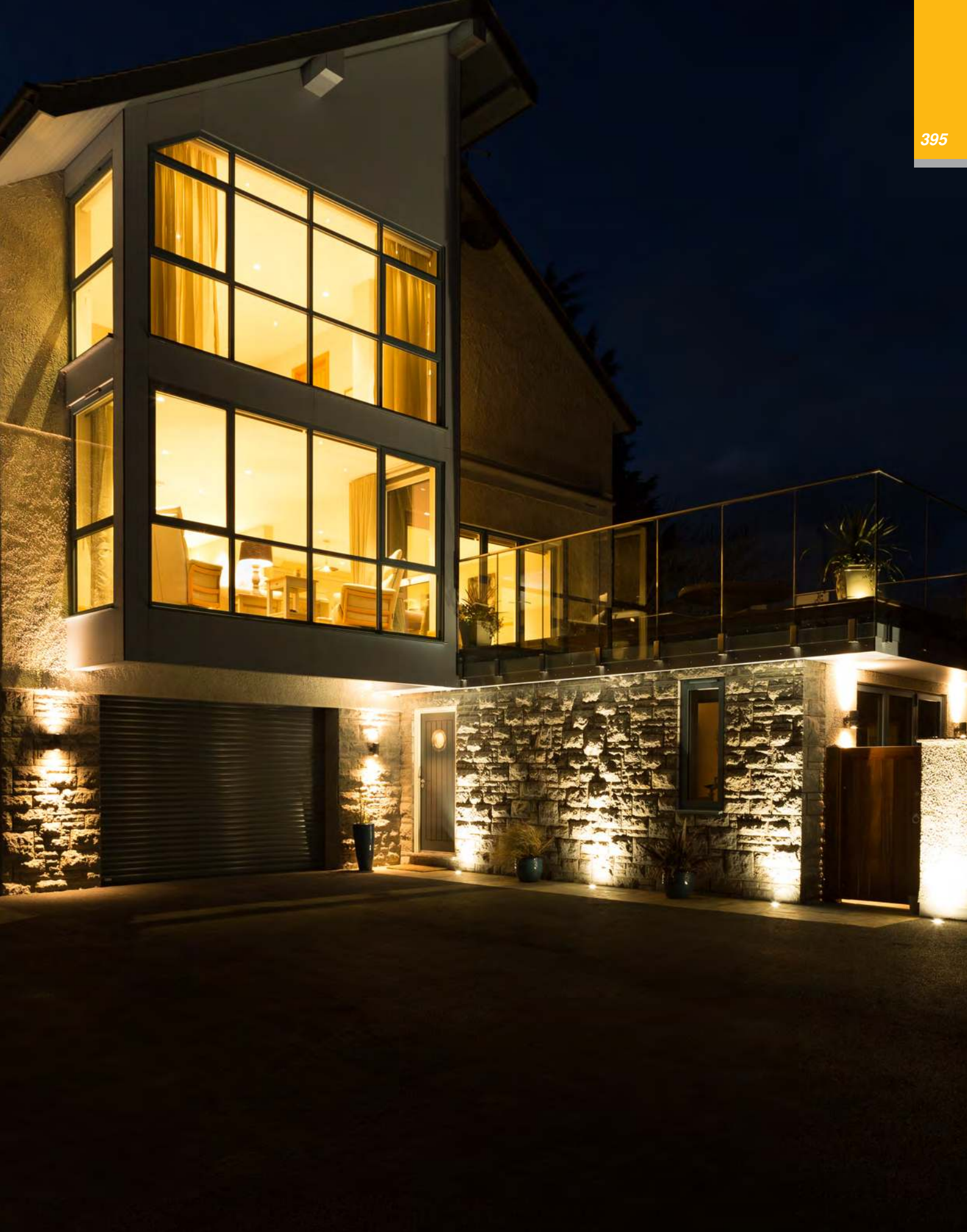
Project - Private Residential Abersoch, UK
